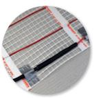
The end joint can be secured in place by taping the red heating element just before the joint to help secure it in place. This will ensure the joint is NOT covered with tape. Both these heating joints MUST now be fully encapsulated within levelling compound and/or tile adhesive.
